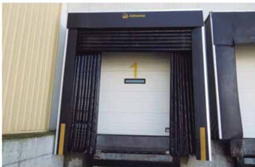
Inflated shelter: it provides a high level of seal.
